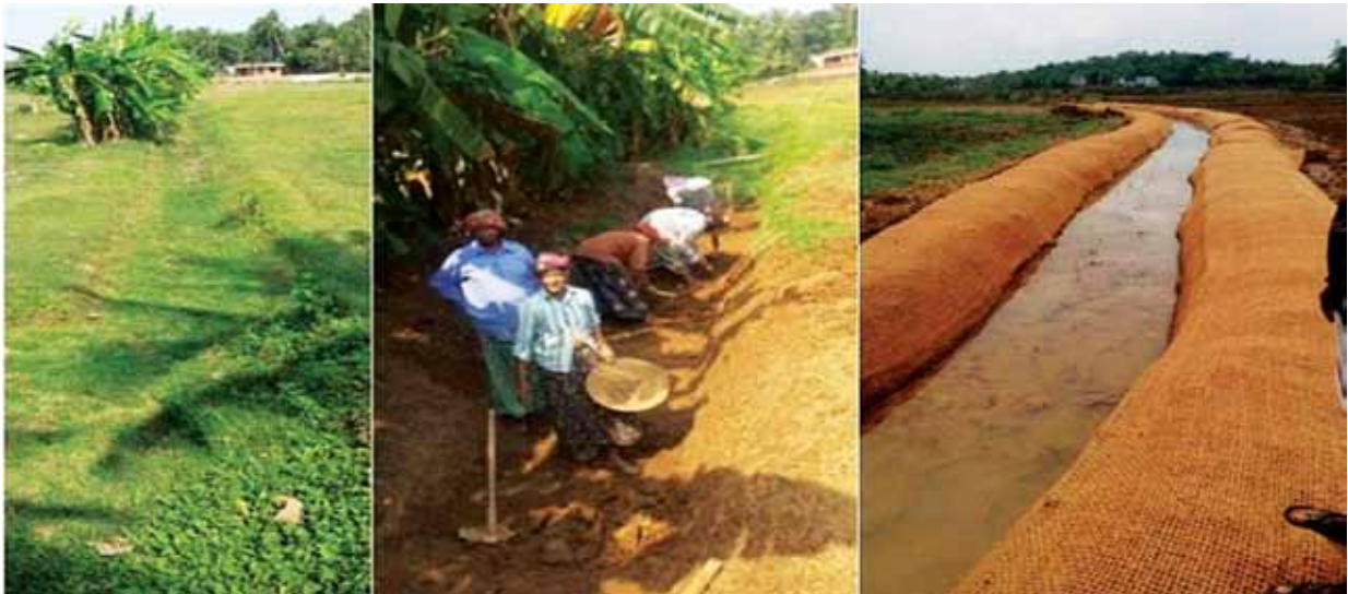
Renovation of traditional water boeies & protection using coir geo textiles-Chirakkal GP
